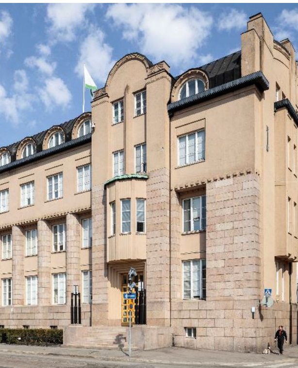
Converting office to hotel at the main railway station in Helsinki, Finland
