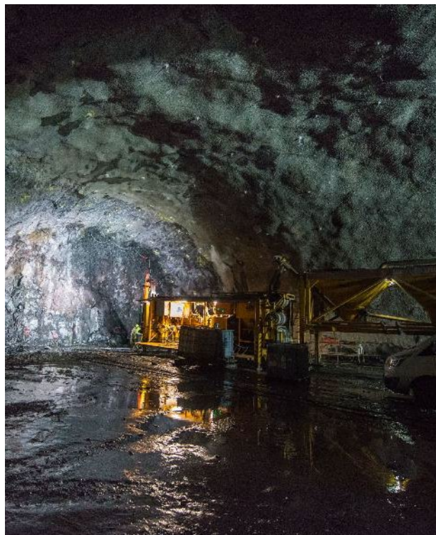
Second tunnel on the Faroe Islands – the Sandøy Tunnel
